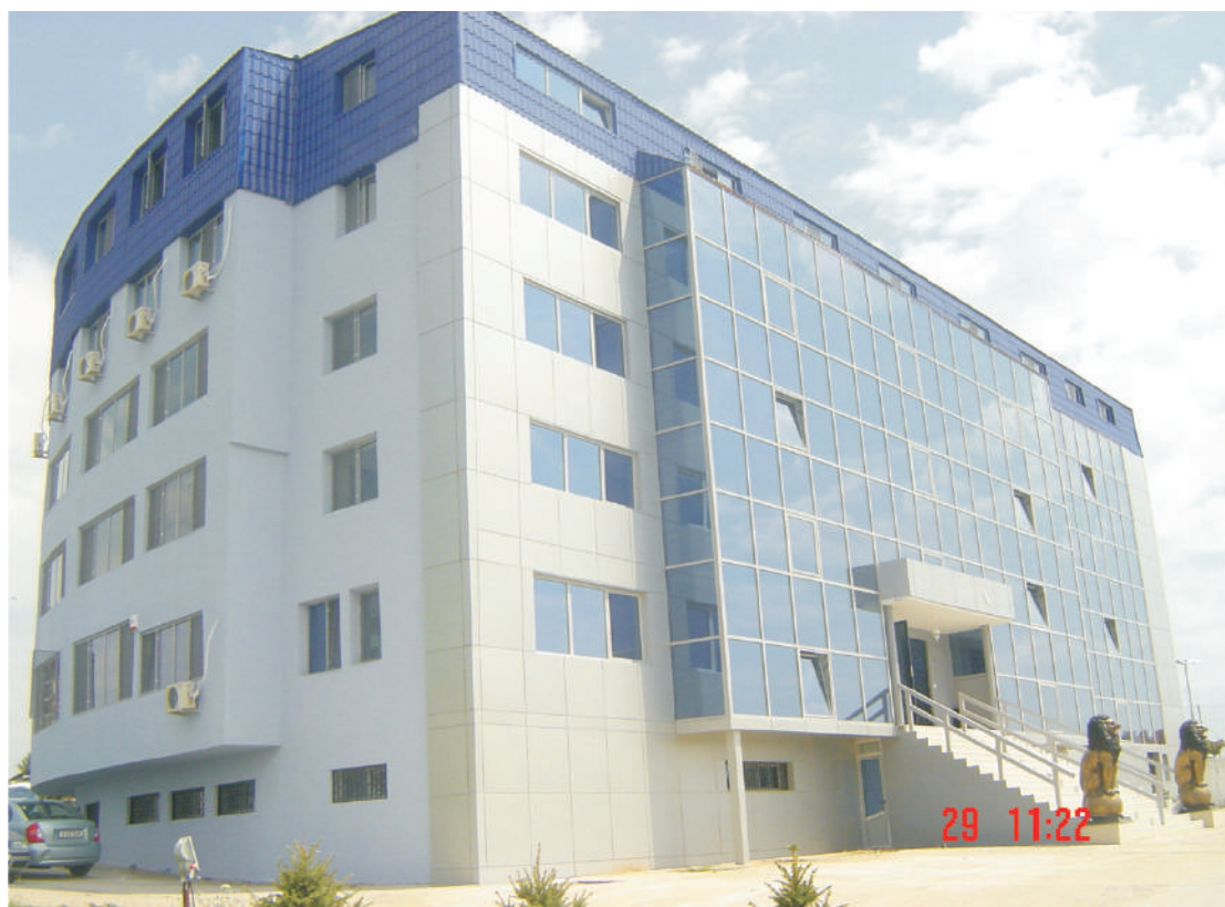
The Bioterra University's administrative headquarters located at meeting of Baneasa Lake and Lake Grivita, united by a stavilar.
